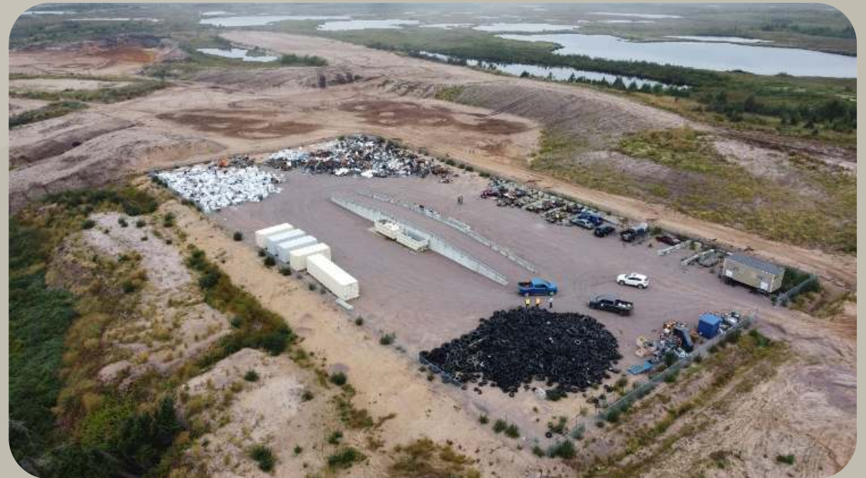
Unamen Shipu Transfer Station
